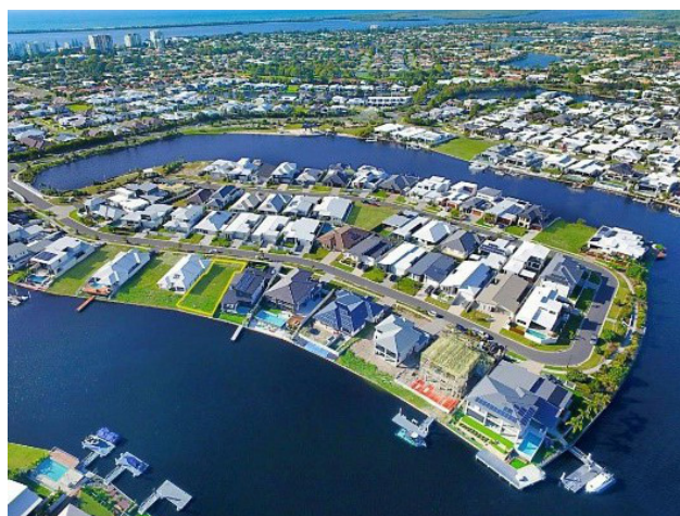
Typical coastal constructed water body development
